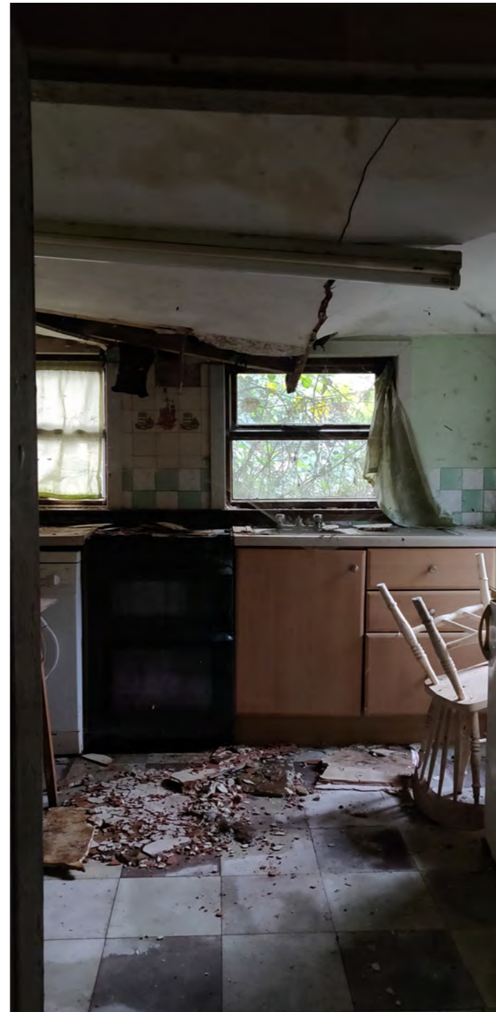
Fig. 10. Photo of rear kitchen annex
