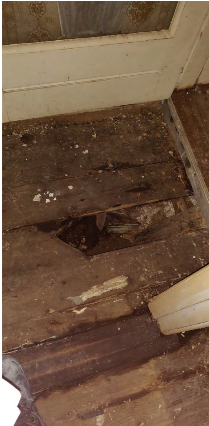
Fig. 4. Photo of suspended timber floor
