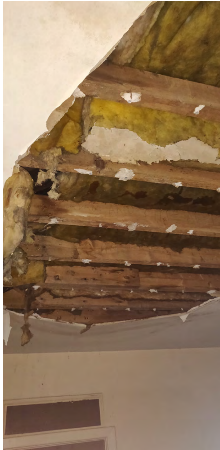
Fig. 5. Photo of living room ceiling
